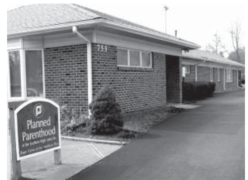
The renovated Elmira health center
